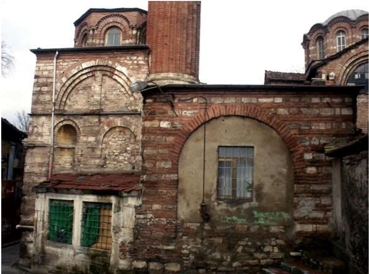
General view from the southwest
