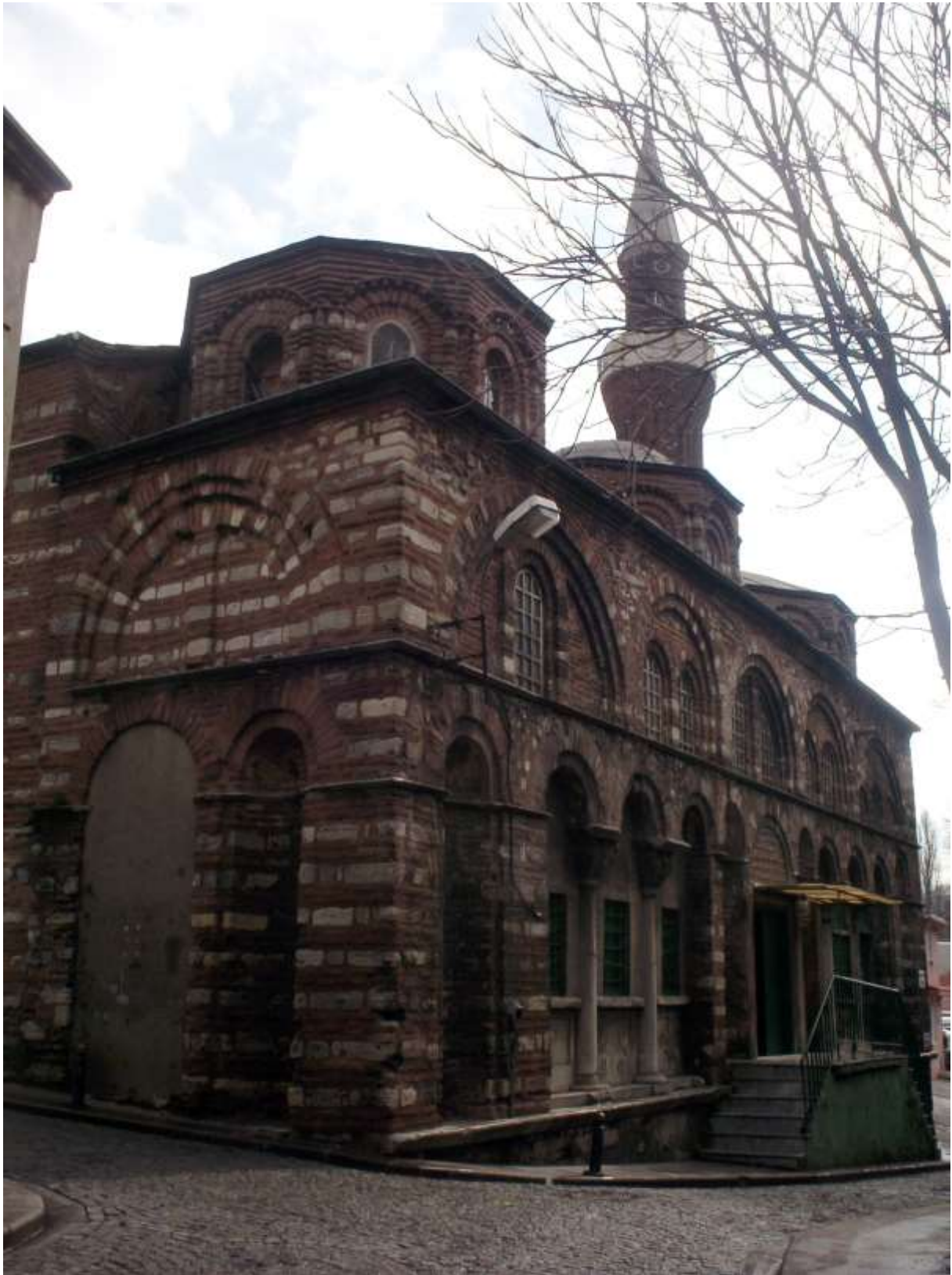
The west façade from the northwest
